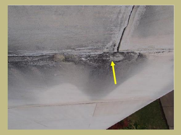
Removal of damaged mortar has been completed.
