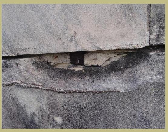
Removal of damaged area is 80% complete. Repair patch work is expected to be completed by end of January.
