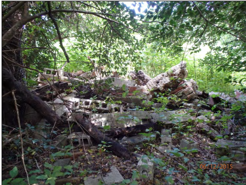
Figure 6-32. Building materials/remnants in a push pile east of the driveway, facing east.
