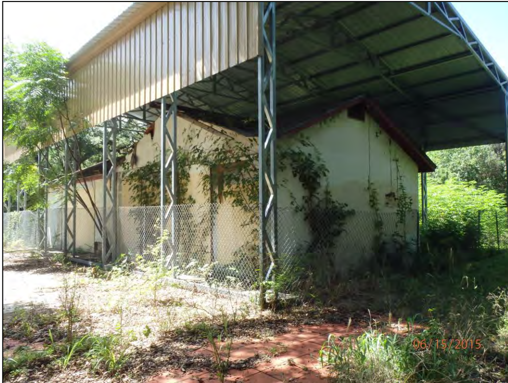
Figure 6-16. Southeast corner of the house, facing northwest.
