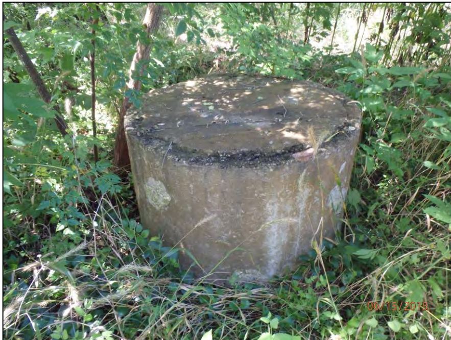
Figure 6-23. Concrete and brick well capped with concrete, facing north.
