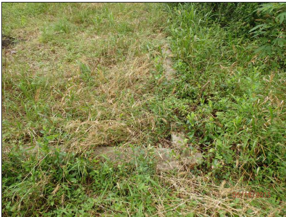
Figure 6-21. Possible concrete foundation south of the patio and house, facing north.
