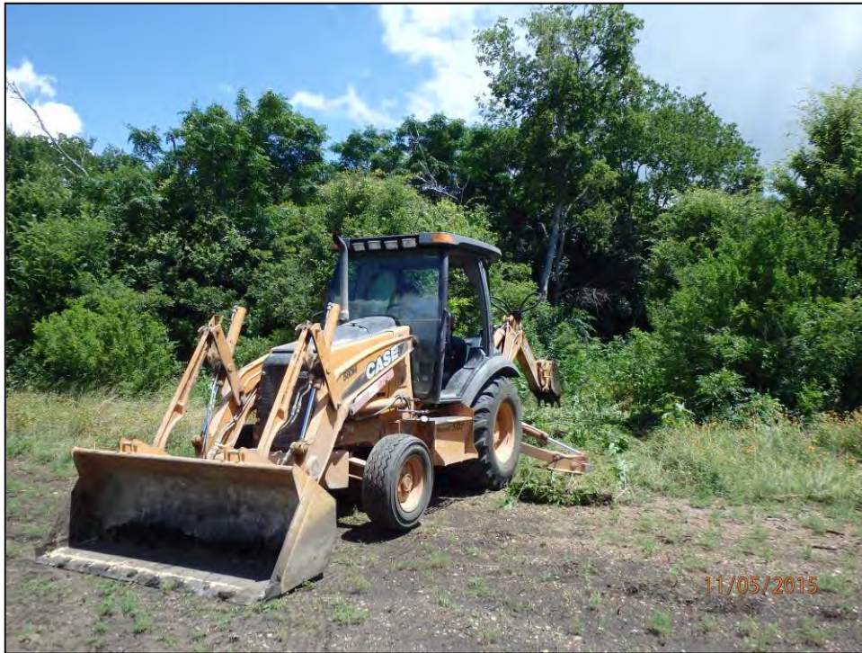
Figure 6-49. Overview of Trench 4 location, facing north.
