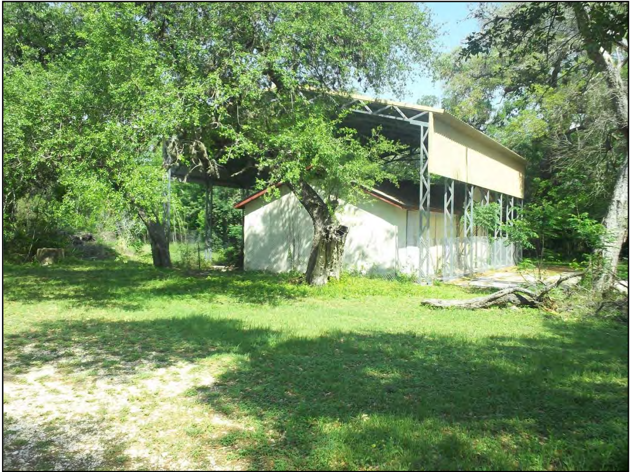
Figure 4-3. Current photograph of the Historic Moses Campbell House.
