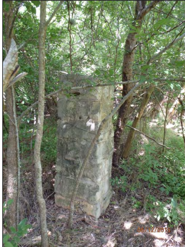
Figure 6-28. Eastern limestone pillar/gate post, facing east.
