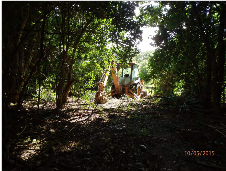
Figure 6-47. Overview of Trench 3 location, facing north.
