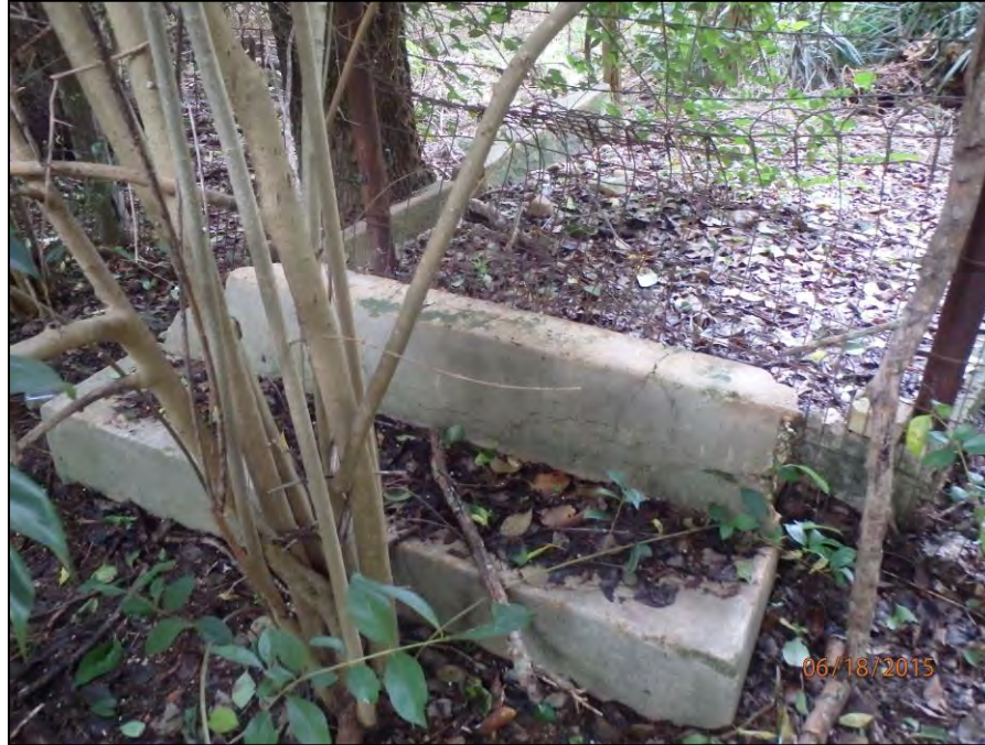
Figure 6-26. Concrete foundation of outbuilding depicted in the 1936 HABS image, facing west.
