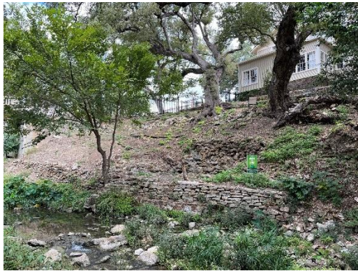
19) East Bank – dry stack limestone chop stone walls
