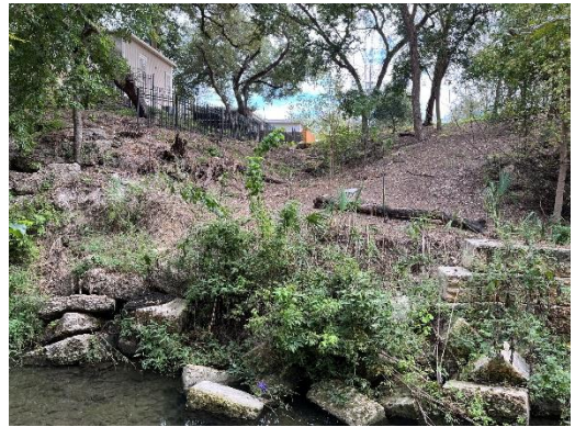
20) East Bank – Upstream failure of 2016 USACE block wall
