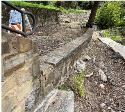
11) East Bank – leaning wall and overbank scour
