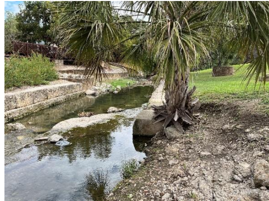
2) West Bank – Flanking by erosion
