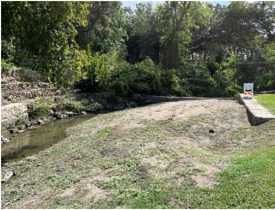
13) Looking downstream (low head dam) – sedimentation
