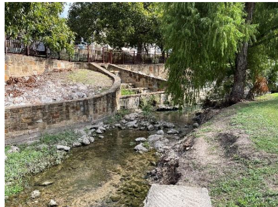
6) West Bank – Minor erosion along unarmored bank
