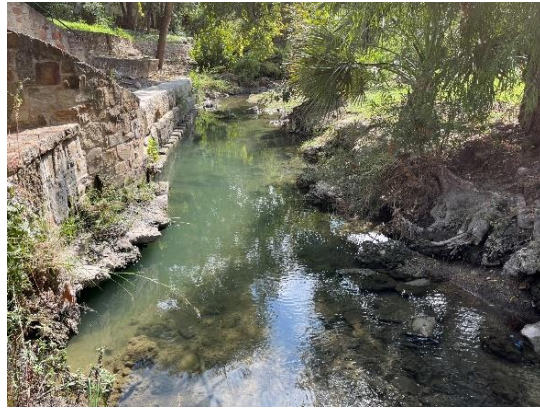
8) Looking downstream – channel downcutting
