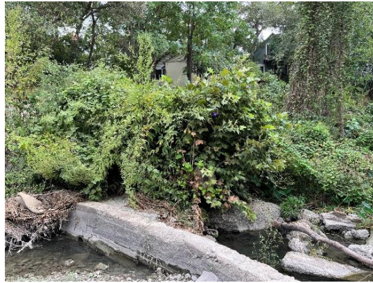
14) East Bank – Flanking of low head dam, sycamore tree root ball failure
