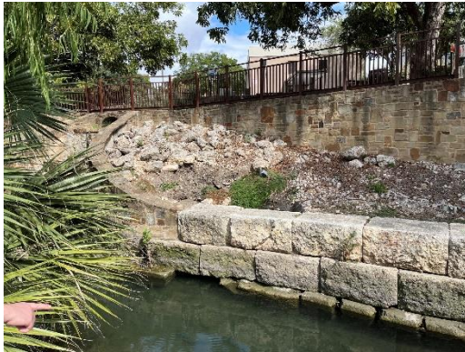
7) East Bank – Missing footer and major scour behind wall
