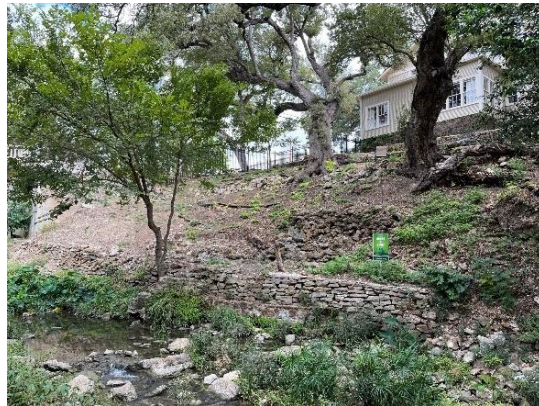
19) East Bank – dry stack limestone chop stone
