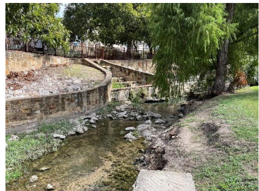
6) West Bank – Minor erosion along unarmored bank
