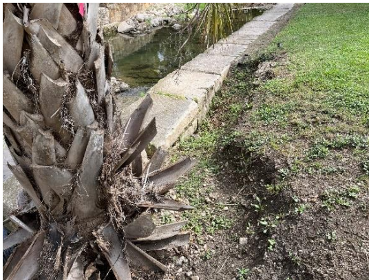
3) West Bank – Erosion behind toe wall
