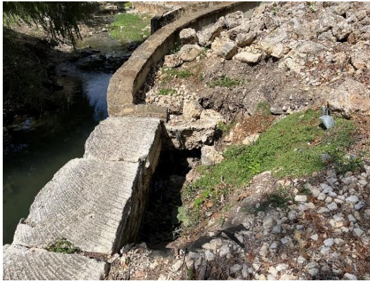
9) East Bank – Loss of backfill behind wall
