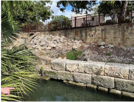
7) East Bank – Missing footer and major scour behind wall
