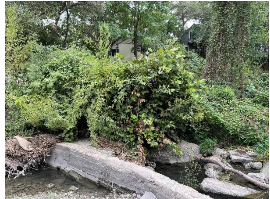
14) East Bank – Flanking of low head dam, sycamore tree root ball failure
