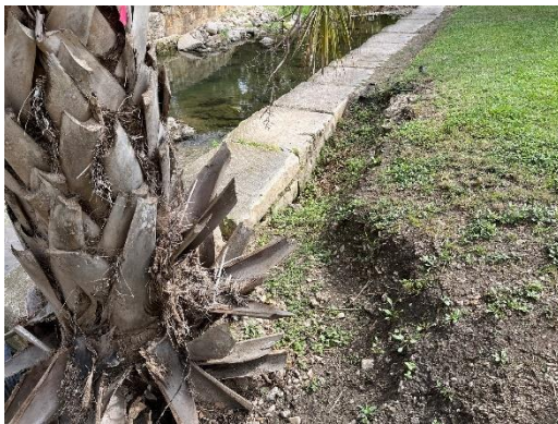
3) West Bank – Erosion behind toe wall
