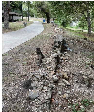
28) West Bank – failed historic stone walls along trail
