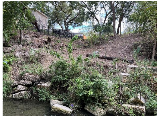
20) East Bank – Upstream failure of 2015 USACE block wall
