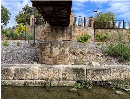
1) East Bank – Bank erosion behind elevated manhole
