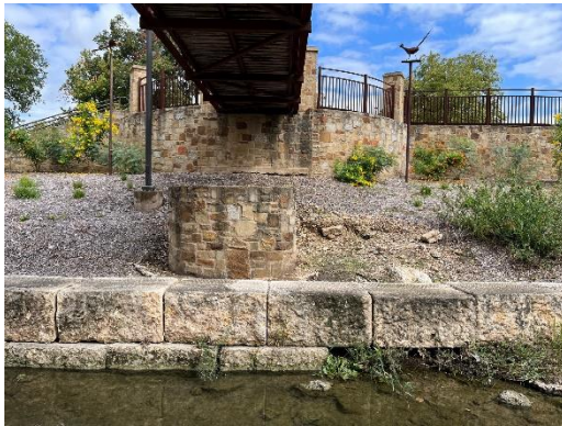
1) East Bank – Bank erosion behind elevated manhole
