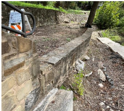
11) East Bank – leaning wall and overbank scour
