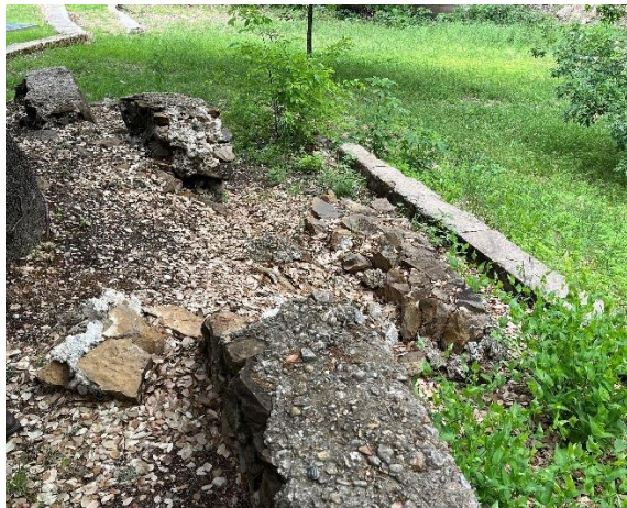
27) West Bank – failed historic stone walls along trail
