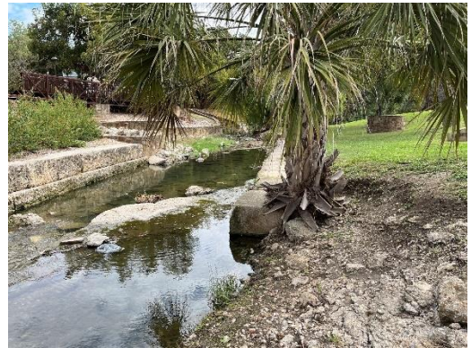
2) West Bank – Flanking by erosion
