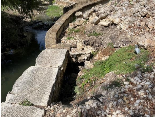
9) East Bank – Loss of backfill behind wall
