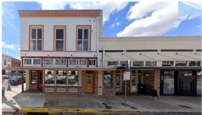
Exhibit 3.11 - South Austin St. - Storefront, Canopies, Windows
