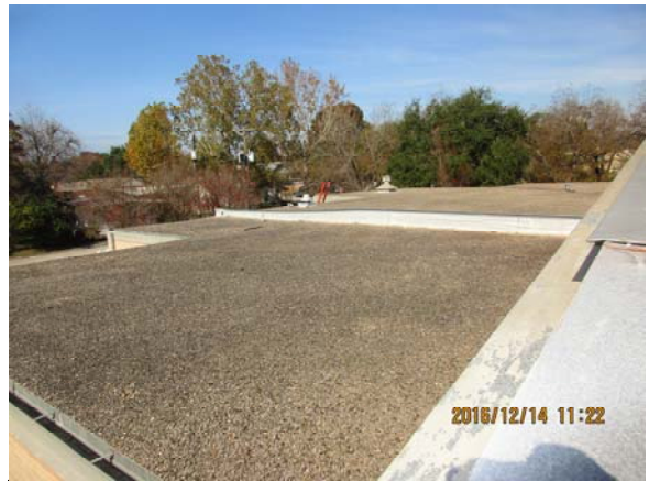
Overview of the roof membrane at the Facility.
