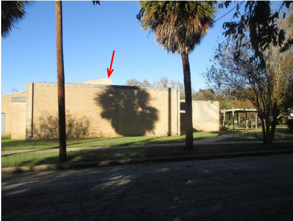
Photo 3: East wall of the Library. One of the three sloping skylights in the 1985 addition can be seen above the roof edge line. The east end of the original building is visible at the right side of the photo.
