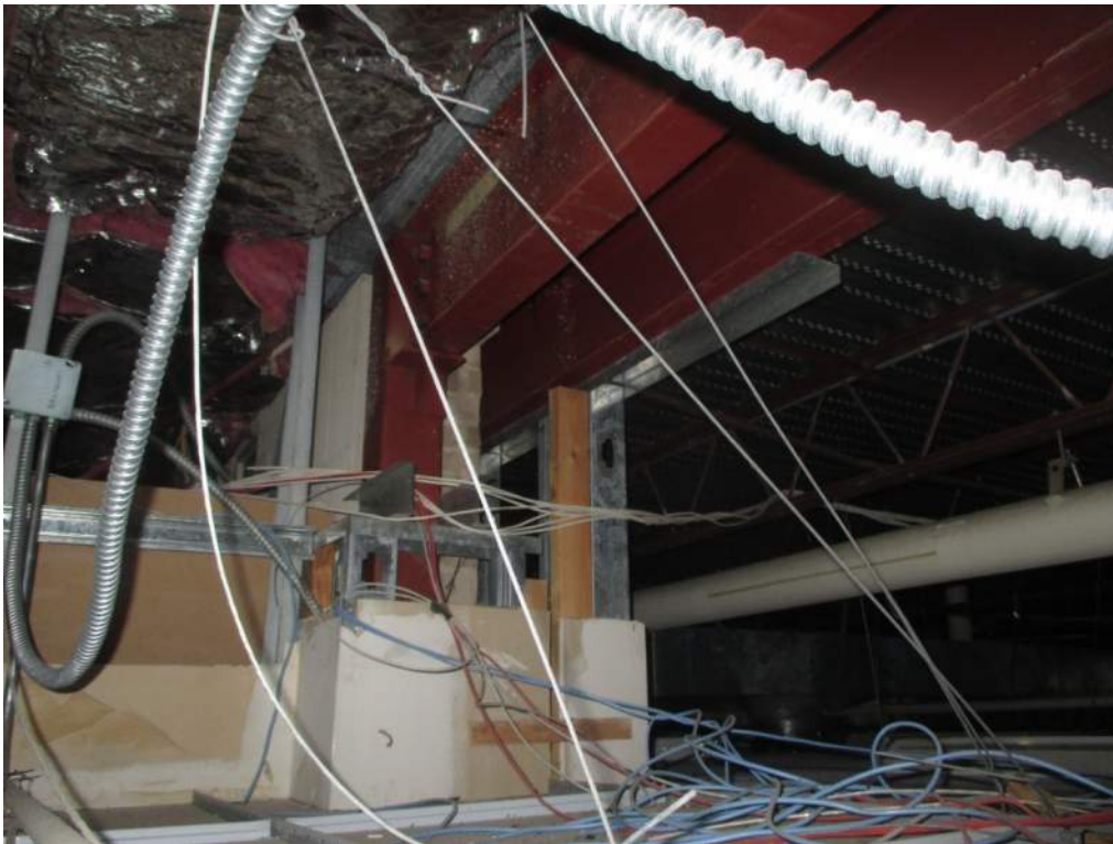
Photo 20: East end of steel beam shown in previous photo, showing new steel column and end of original load bearing CMU wall at connection between original building and addition. Note brick was the original south exterior wall.
