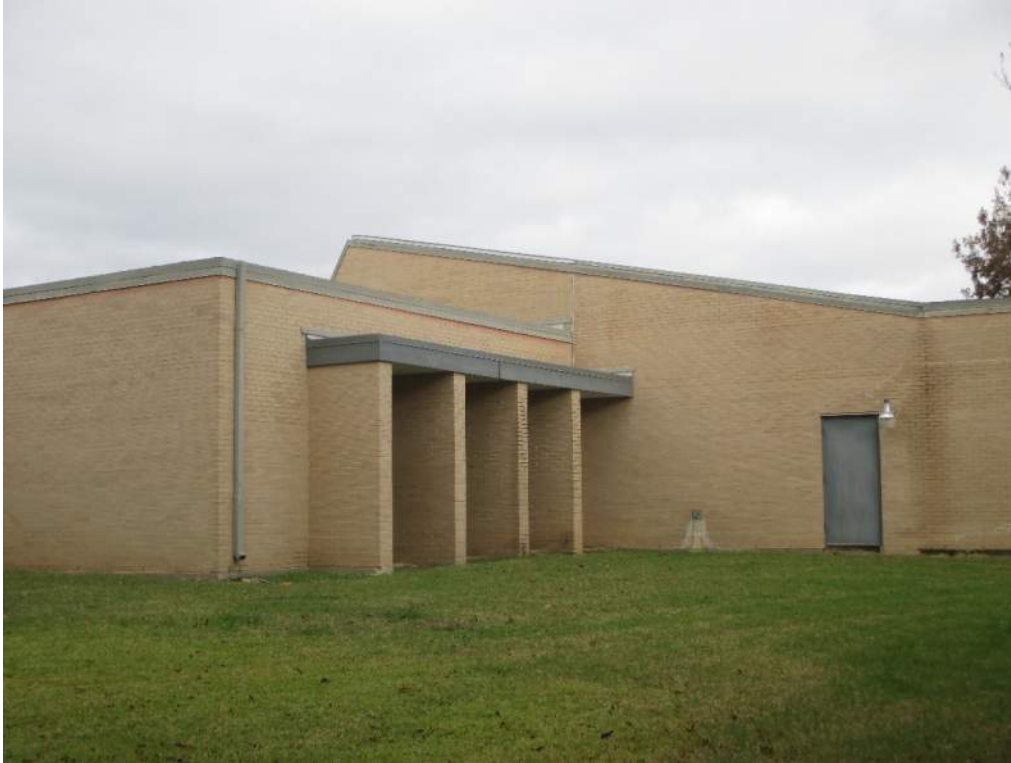
Photo 13: West side of 1985 Addition showing sloped roof/wall at skylight. Note expansion joint in brick at reentrant building corner.
