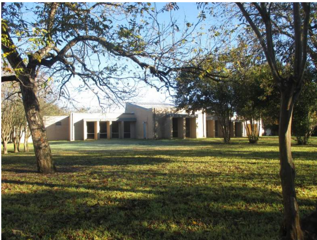
Photo 6: South face of building addition showing sloping roof over clerestory skylights.
