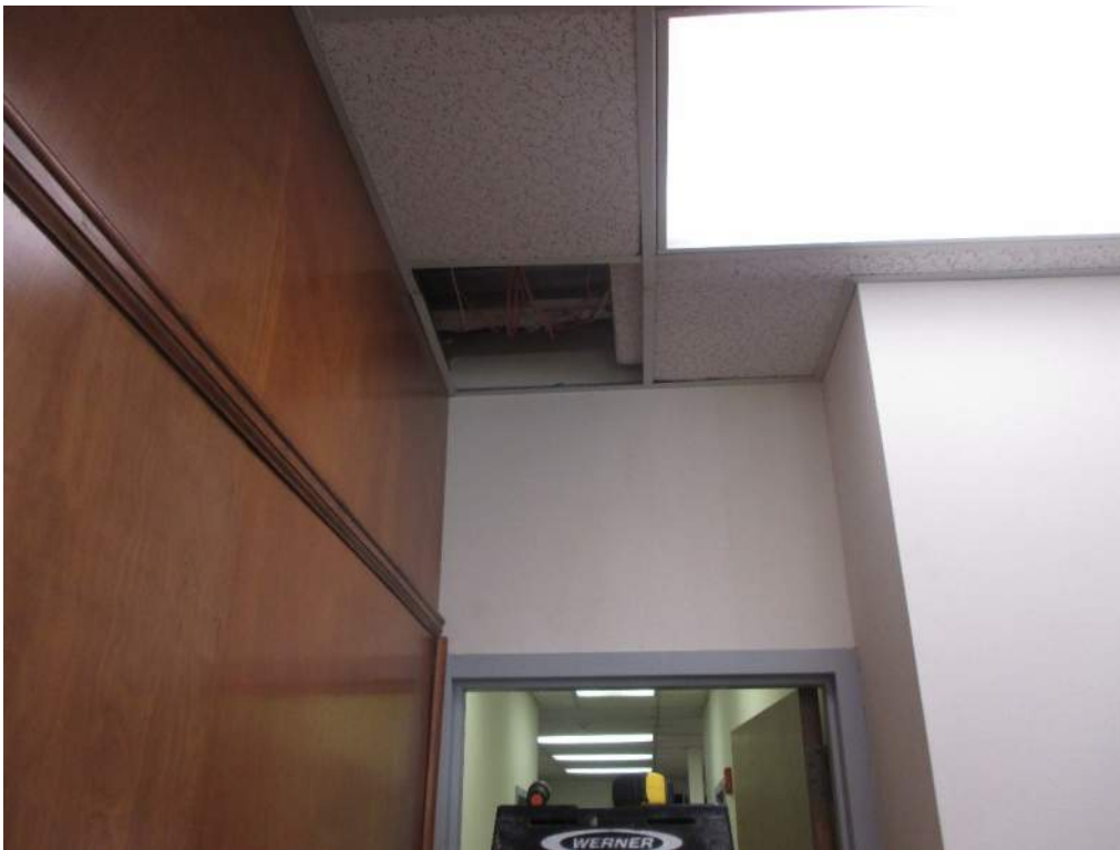
Photo 26: View looking north into the administrative office area of the original building from the Addition. The original load bearing CMU wall and brick veneer were cut through at this location in the 1985 Addition work.
