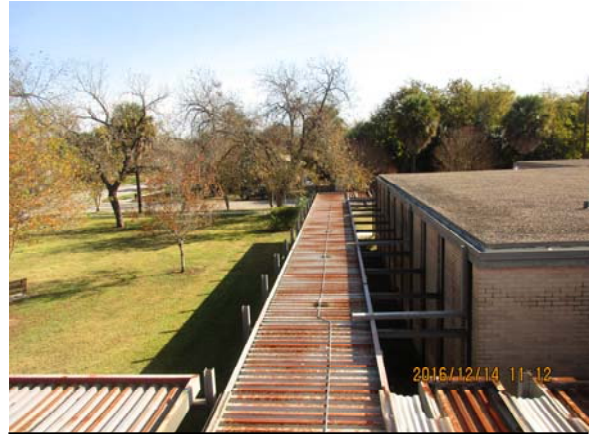
Overview of covered canopy walkways.
