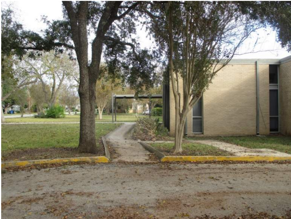
Photo 2: Exterior view looking east along the original front of the building showing potentially poor drainage in this area. The front canopy is visible in this photograph.
