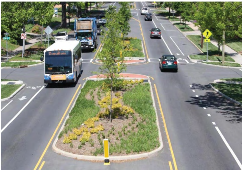
FIGURE 14: RAISED MEDIAN EXAMPLE
