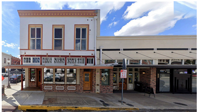
Exhibit 3.11 - South Austin St. - Storefront, Canopies, Windows
