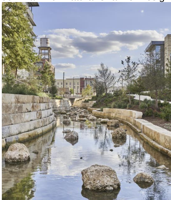
Figure 3: Limestone Block Wall Example
