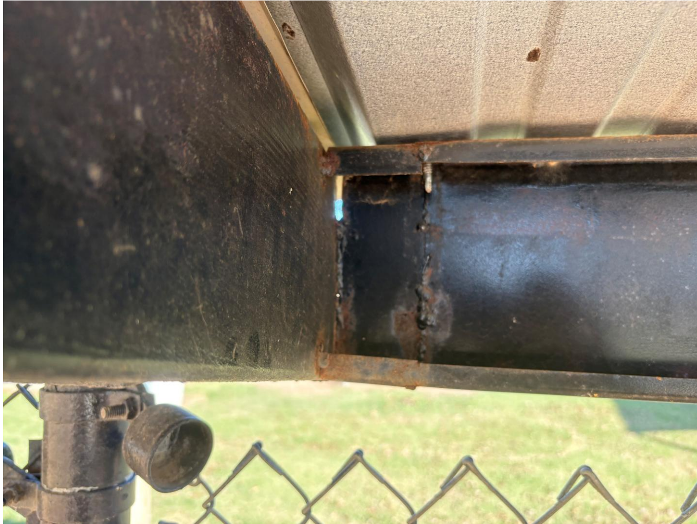
Image 3: Dugout Roof Damage, Severe
